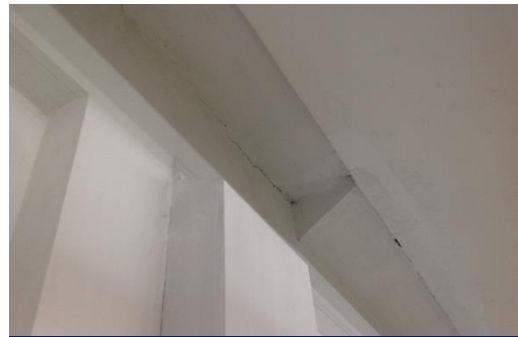
Cracking at slab interface
