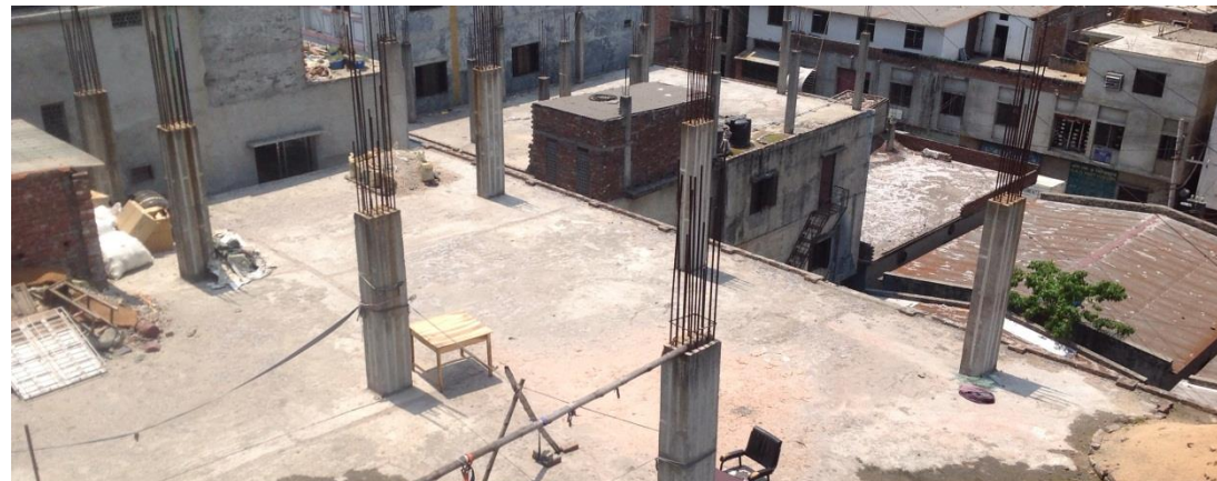
Lower Roof Parapet
