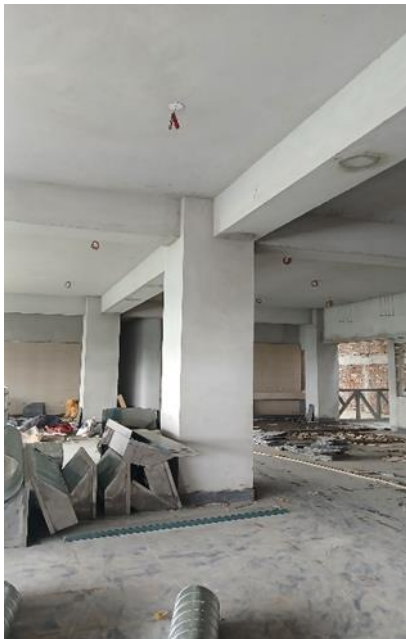
Beam column frame
