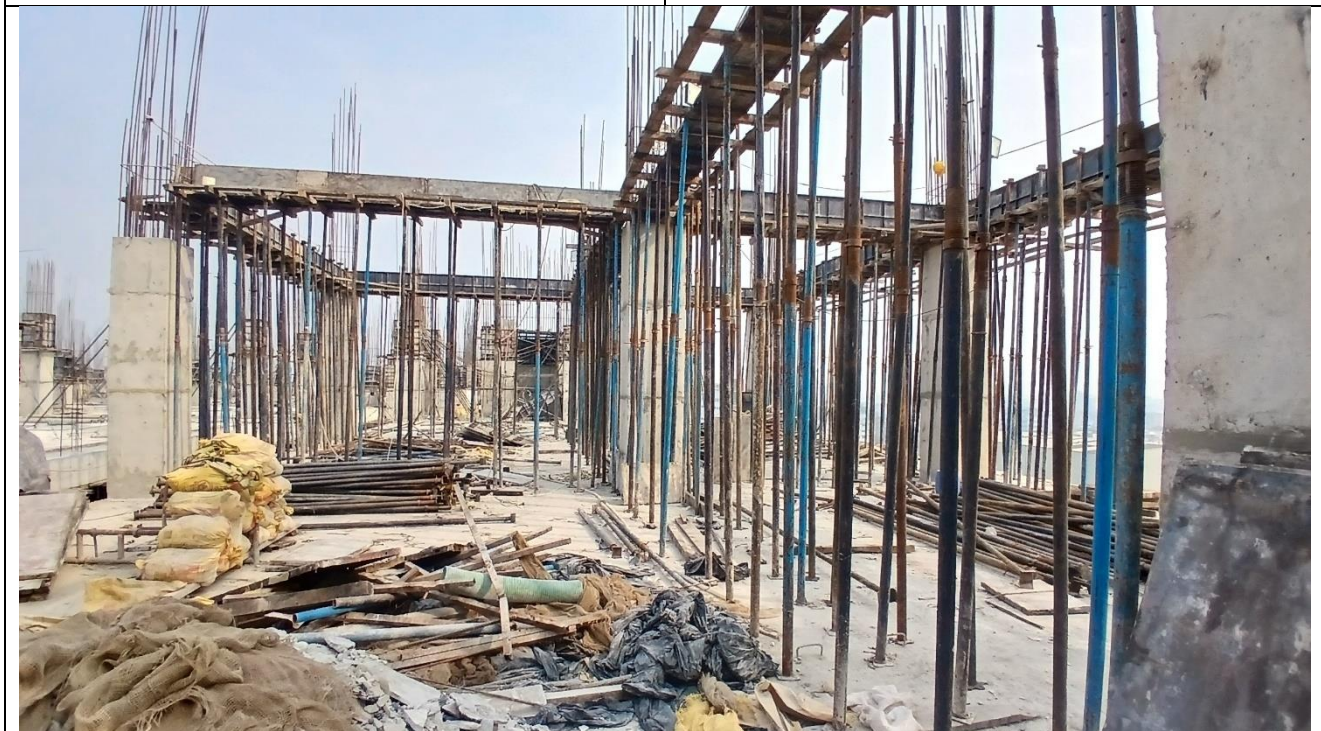
Existing Roof (7 th Floor)
