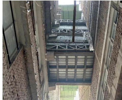
Connecting bridge between two building
