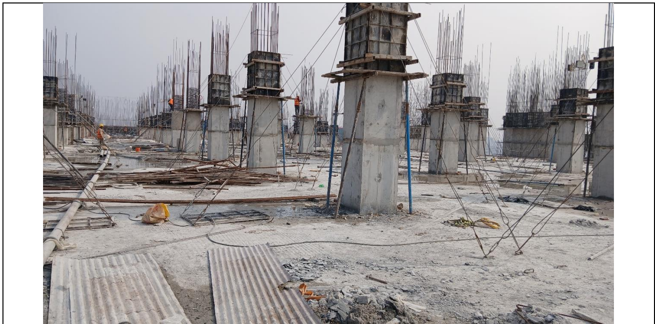
Existing Roof (7 th floor)
