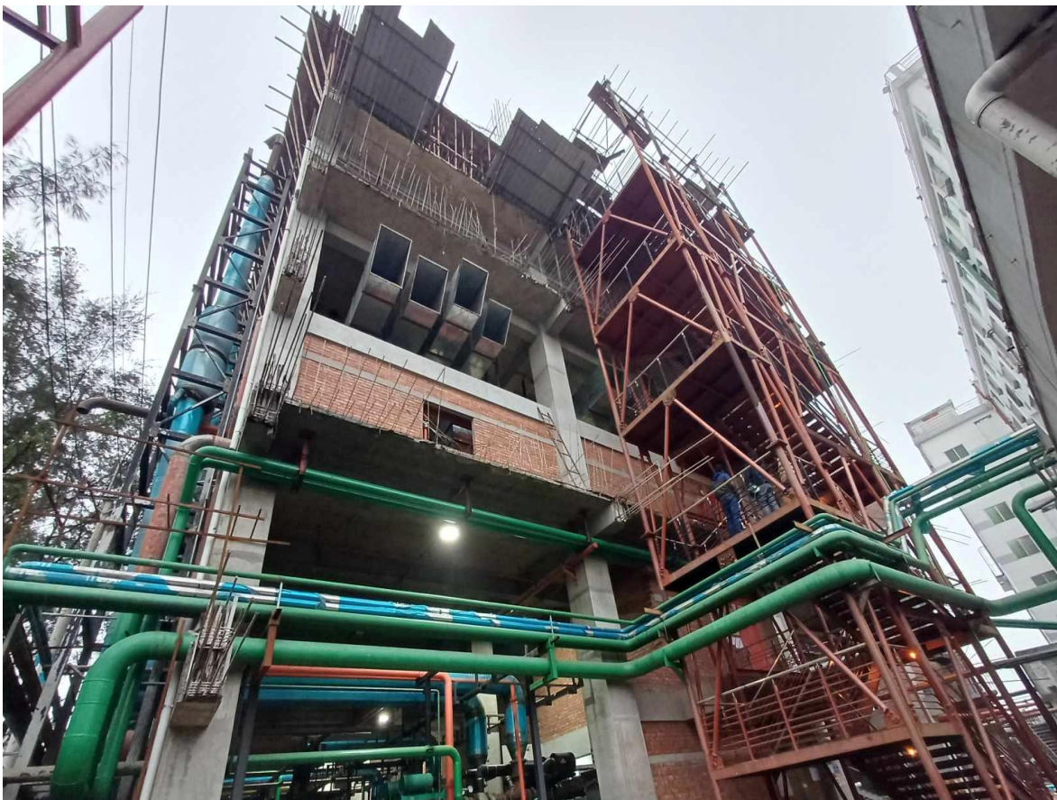
Beam-slab re-bar kept exposed for future horizontal expansion
