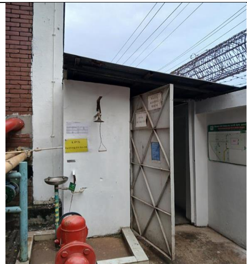
Building-12: Wastage Store Shed
