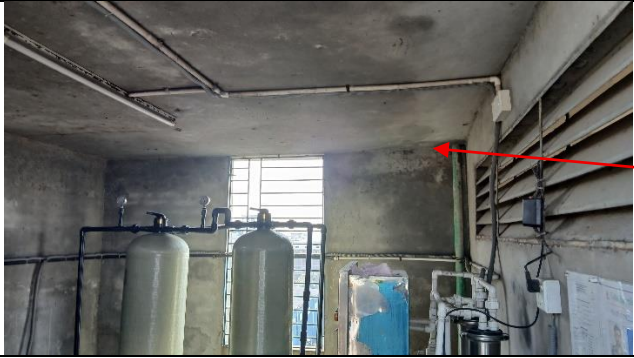
Missing cantilever beam on stair roof
