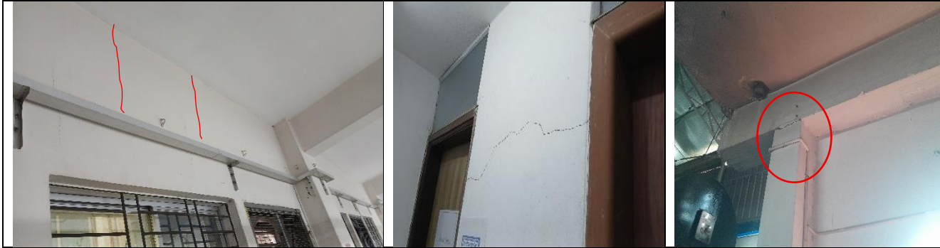
Periphery brick wall Internal brick wall Boiler Room
