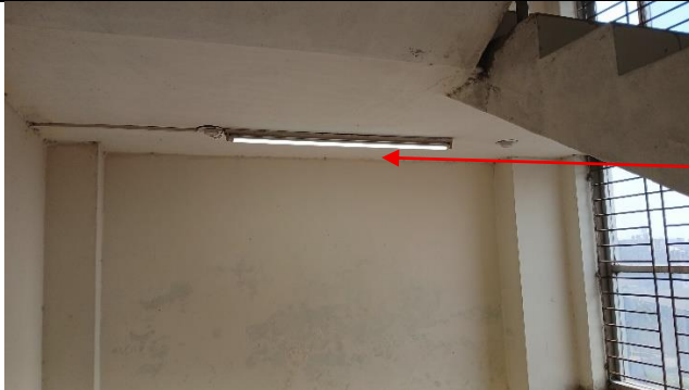
Missing landing beam on stair zone.
