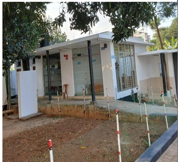
Fire Control & Security Room
