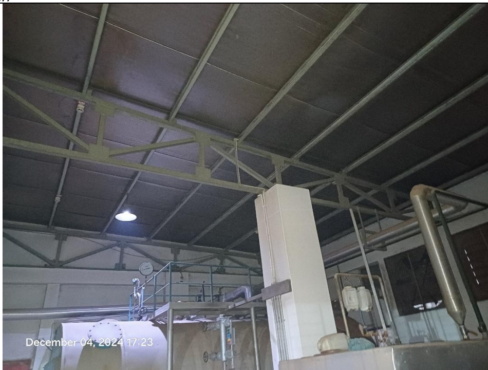
Truss in North-South direction
