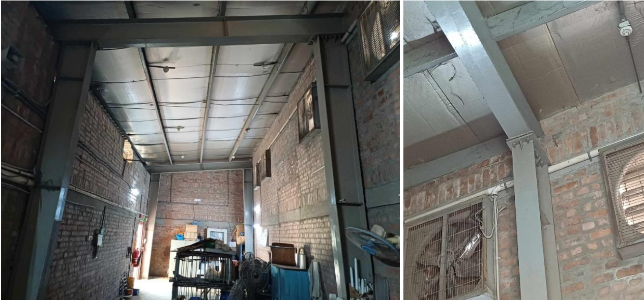
No lateral load transfer media in long direction
