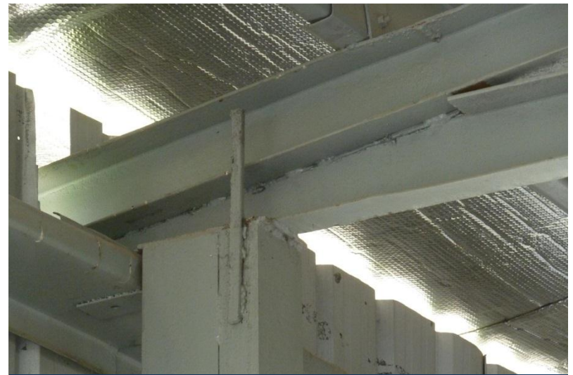
Truss supported on box section column, fabricated from individual sections
