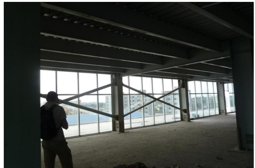
Cross bracing to end bay
