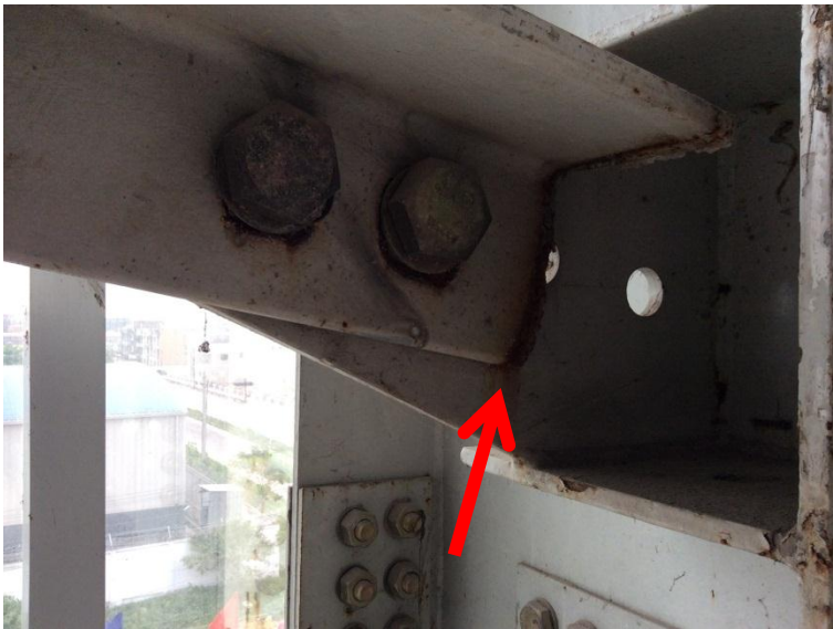
Example of modified cross bracing connection
