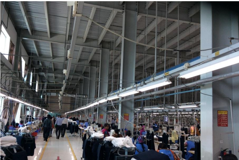
Primary structure seen from Ground Floor
