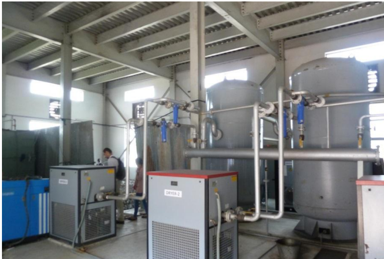
Primary structure seen at Ground Floor
