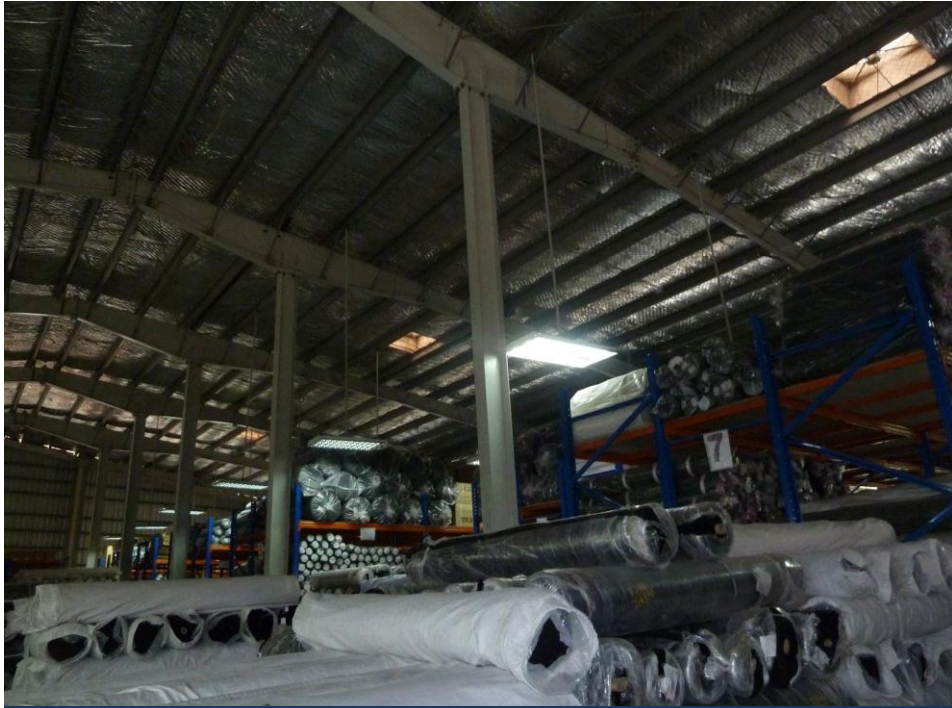
Portal Frames seen from building interior
