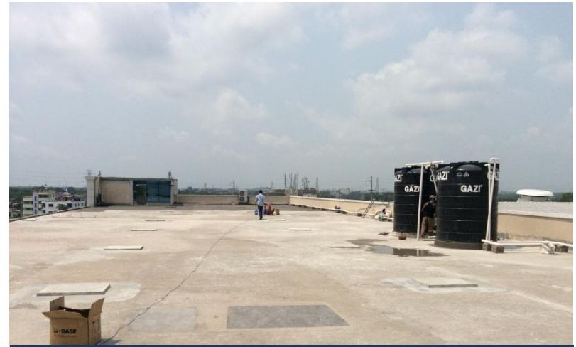
Reinforced concrete roof at east end of Building 1
