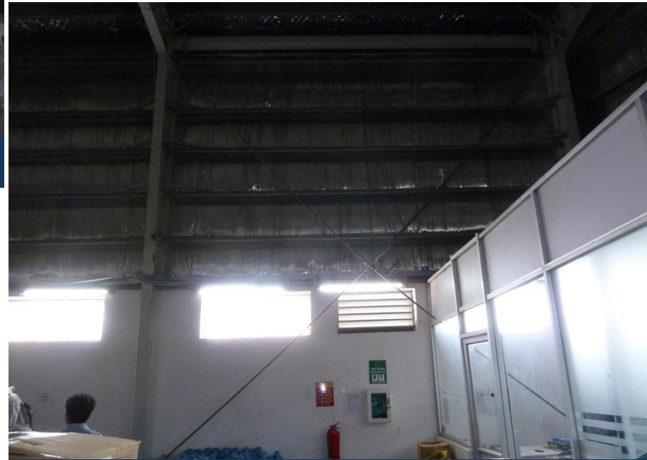
Example cross bracing in building side wall
