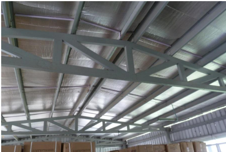
Trusses to part B
