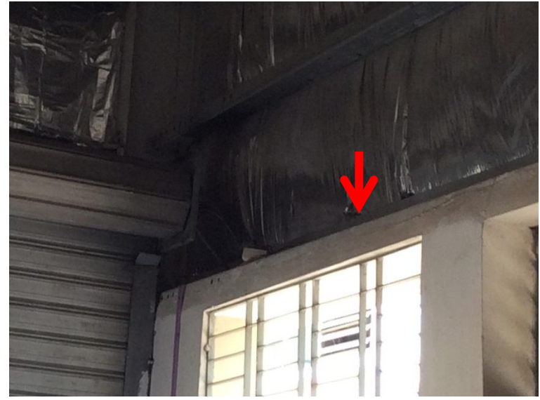
As constructed, lateral support to tops of brick walls is not clearly defined
