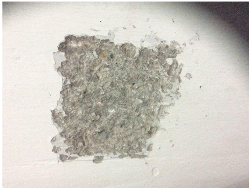
Tested Basement Floor Column – Stone Chips
