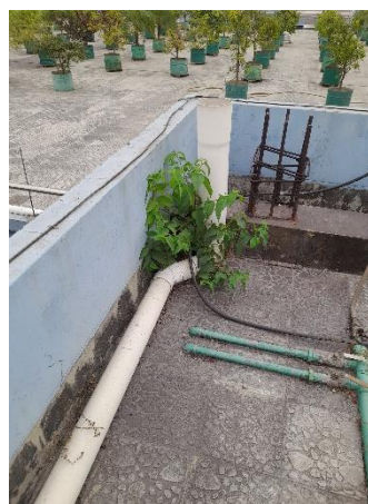
Exposed re-bar and vegetation at roof
