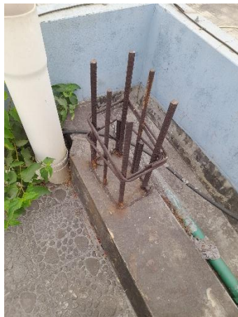
Exposed re-bar and vegetation at roof
