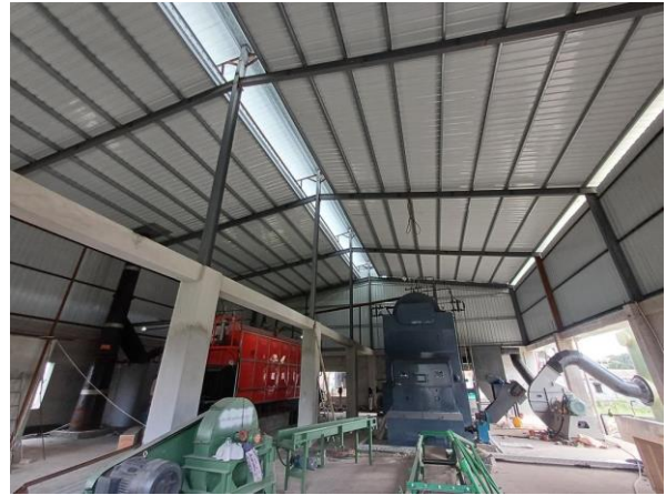
Jhut Boiler Shed
