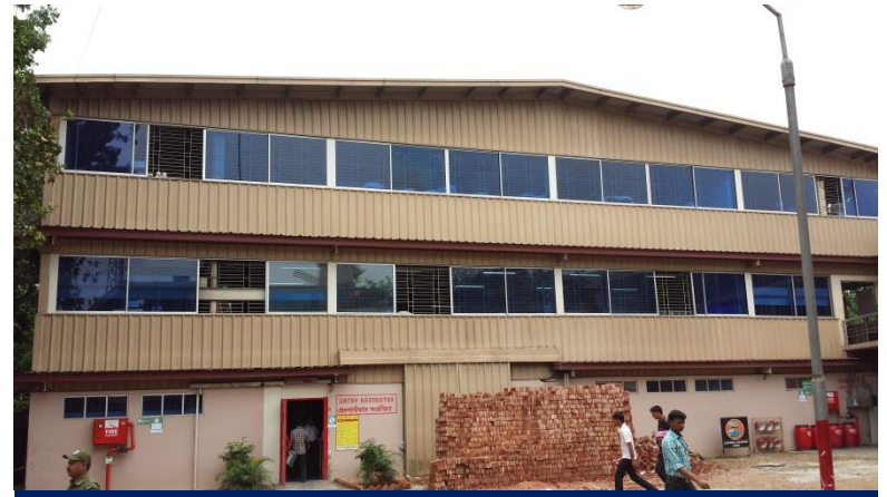
Front (north) elevation of Production Bldg #2
