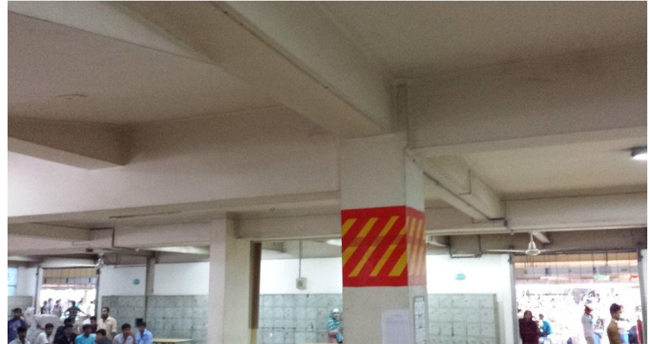
Concrete beam-columns frame system
