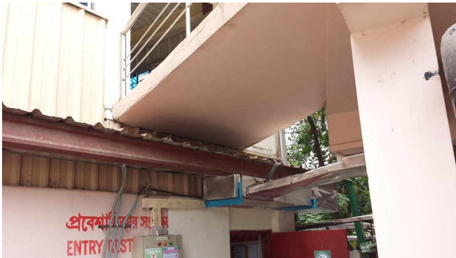
Linking bridge between Production bldgs
