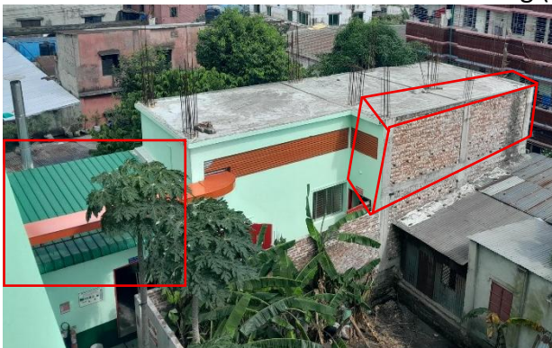
Undocumented column and extended portion
