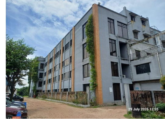
Building-2: New Production Building
