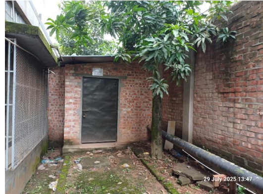
Shed-7: RMS Room
