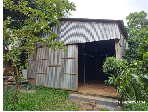
Shed-3: Jhut store
