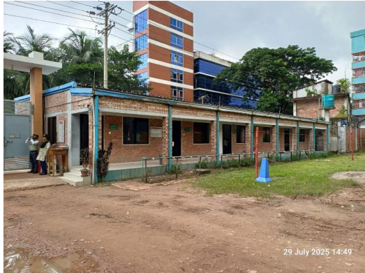
Shed-5: Security Shed
