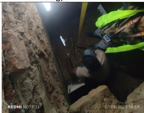
Figure 12: Footing top is 70 inches from PL at the edge.
