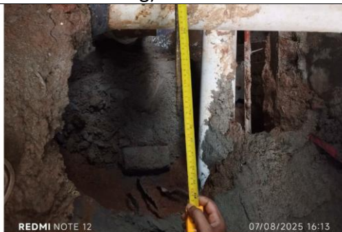
Figure 29: Footing thickness is 18 inches at edge.
