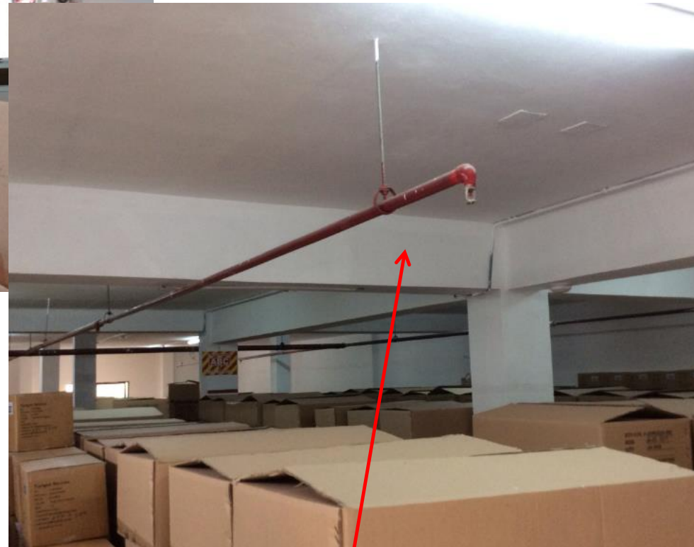
Beams and Slab on underside of 1 st and 2 nd Floors
