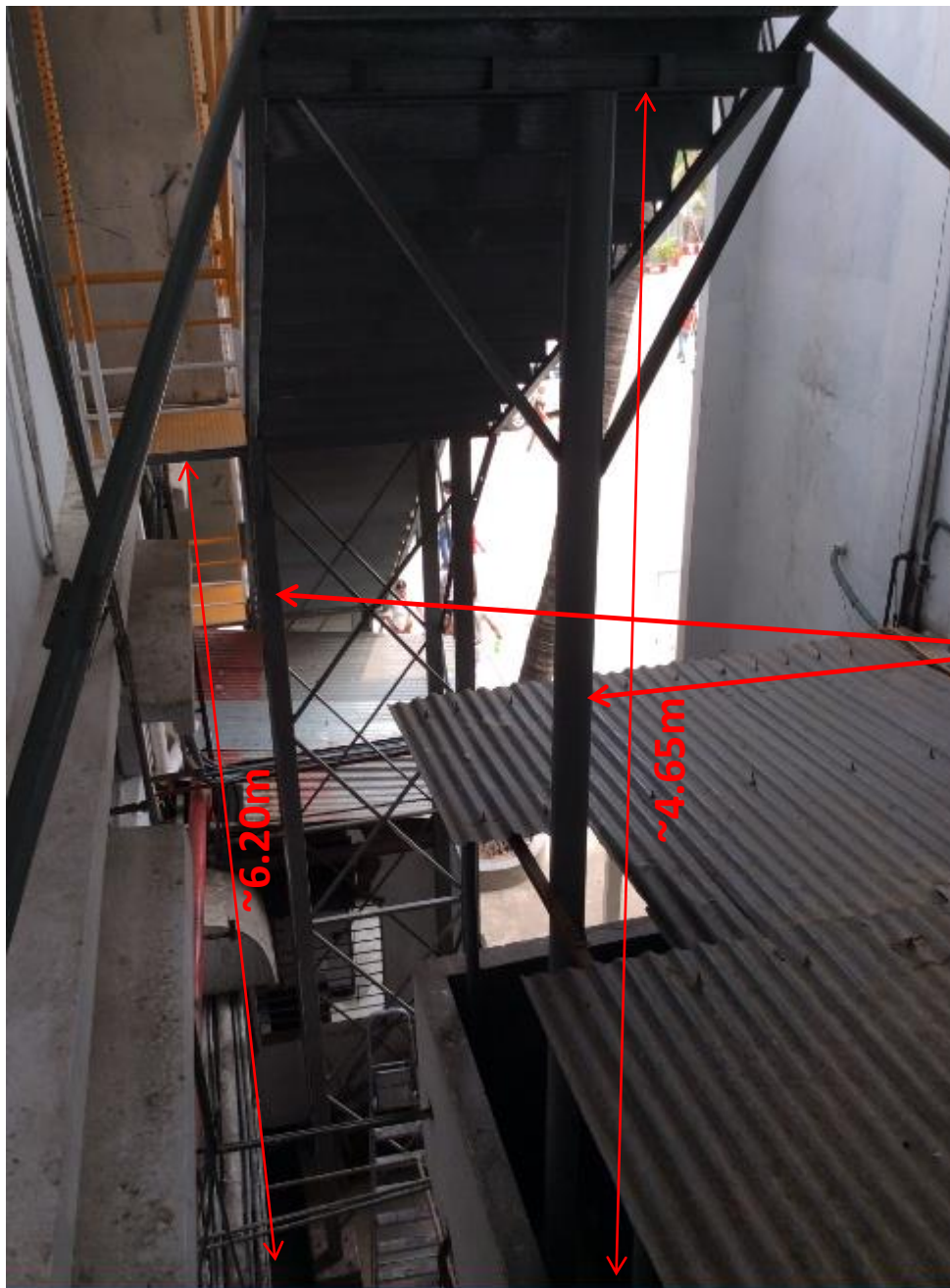
Slender Columns Supporting Steel Stairs
