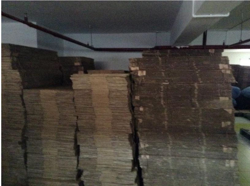
Heavy loading observed on 1 st floor
