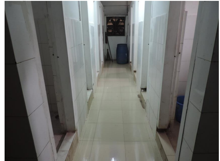
Toilet built up in the marked area
