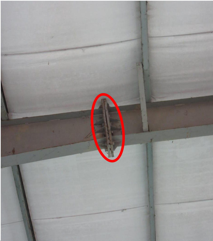
Gaps between End Plates of Frame Beam Splice Connections
