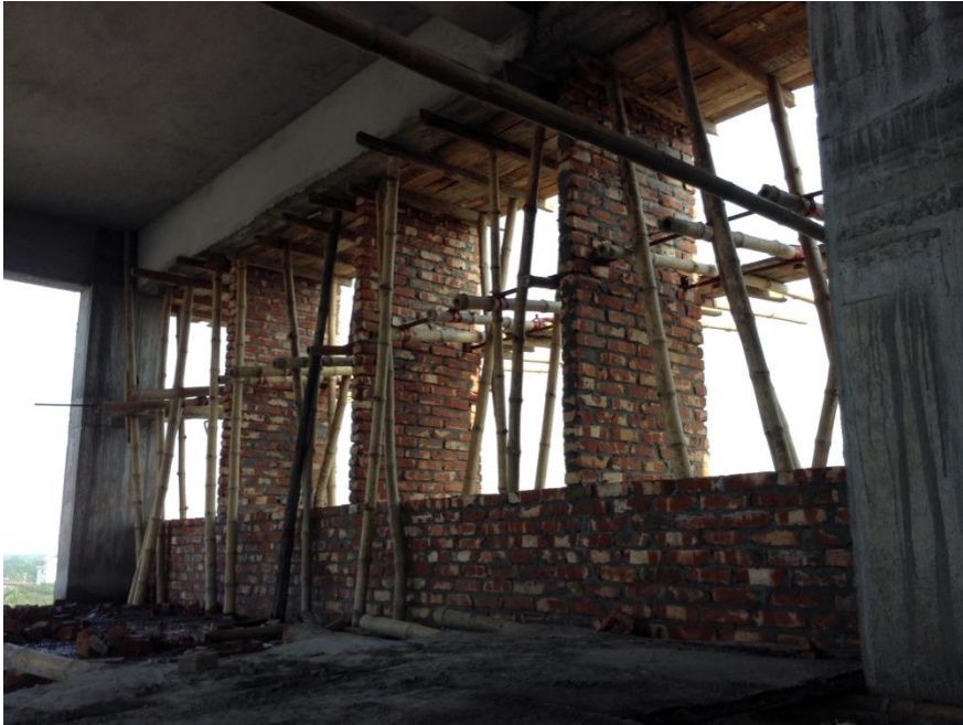
Façade wall with brickwork fins unrestrained over 3.67m floor-to-ceiling height force
