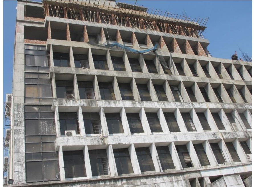
Façade wall with brickwork fins unrestrained over 3.67m floor-to-ceiling height force
