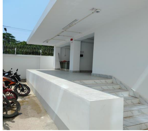
Security & Fire Pump Room
