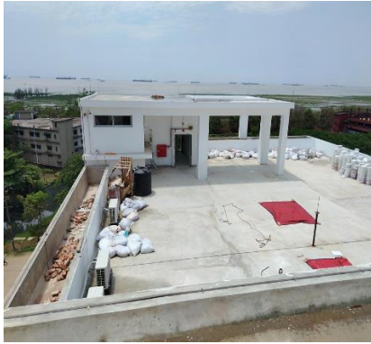
Additional brick wall & build-up for roof gardening provision
