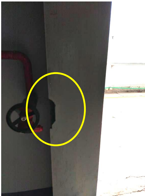
Cut off the flange in the steel column
