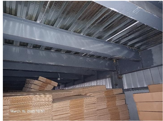
Secondary beam of the mezzanine
