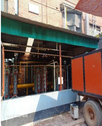
CNG Plant Shed
