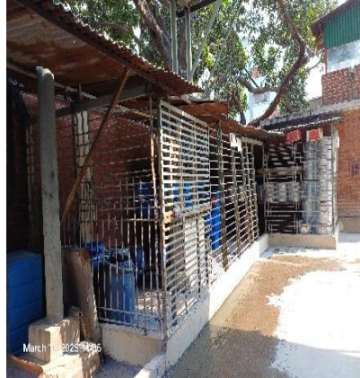
Empty drum shed
