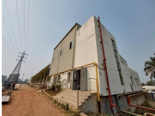
Building-7: HTL- 2 Utility Building
