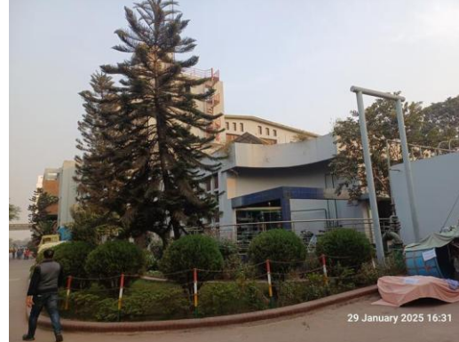
Building-8: WTP Building- 1
