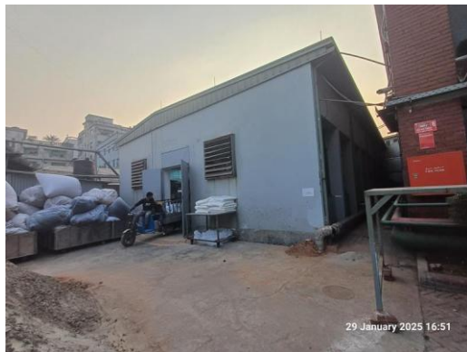
Building-11: Acid Wash Shed
