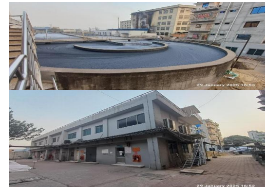
Building-9: ETP -1 & Building-10: ETP Monitoring Building-1
