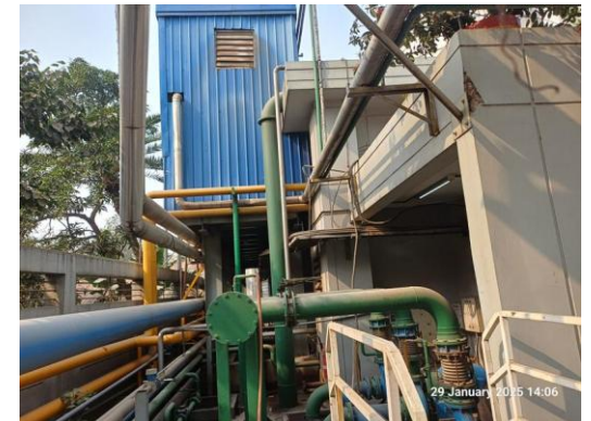
Building-13: EGB Shed-1
