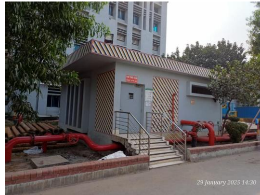
Building-12: Fire Pump Room
