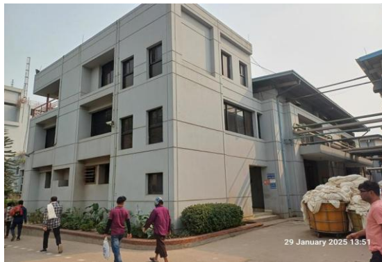
Building-4: Boiler & Compressor Shed (Hamza-1)
