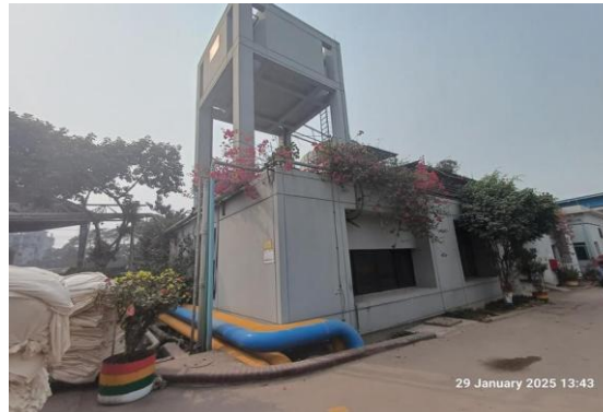
Building-5: Generator & Power Control Building (Hamza-1)
