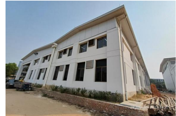
Building-3: Washing Production Building With Shed
