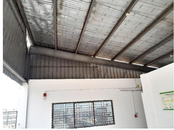
Roof shed above stair at south-east corner
