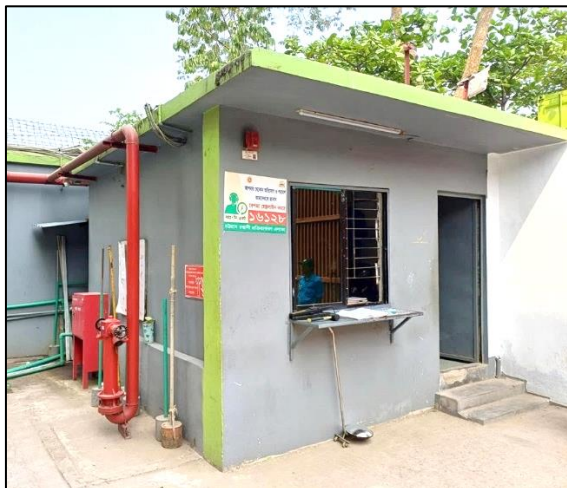
Security Building & Fire Command Room
