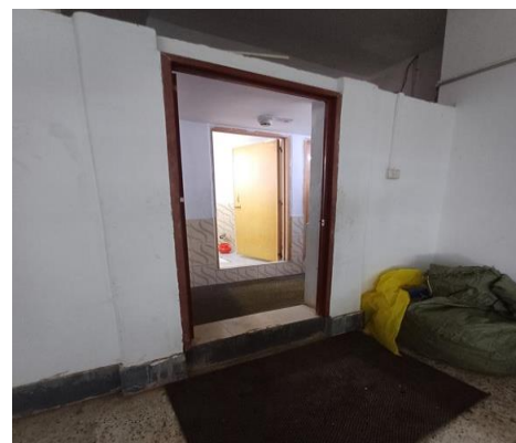
Build-up & false slab t toilet area
