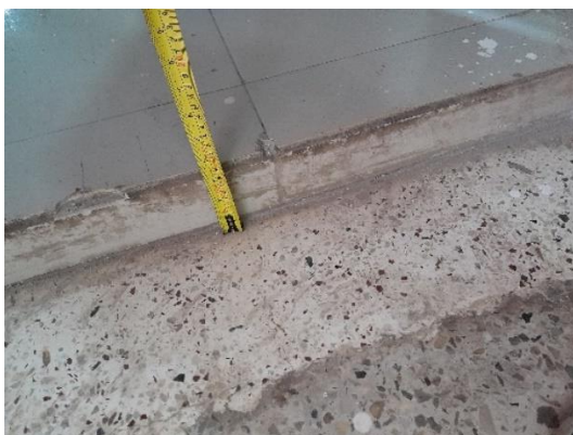
Build-up at 5th floor dining
