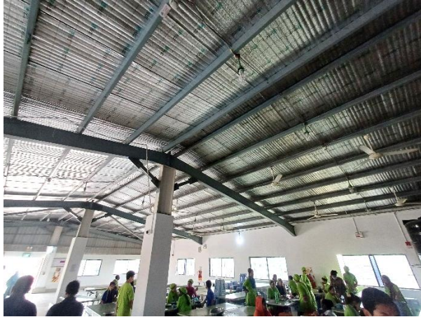
Roof Shed above 5th floor dining
