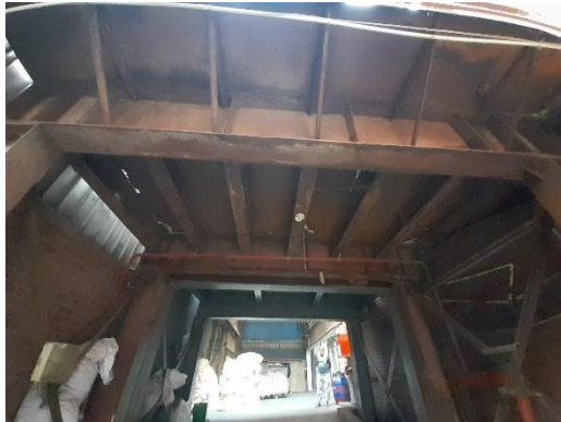
Corrosion on steel member of steel stair
