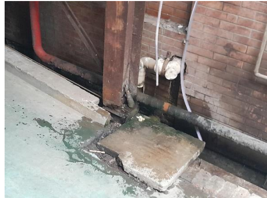
Corrosion on steel member of steel stair
