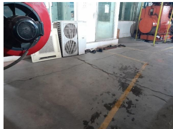
Crack on Ground floor slab
