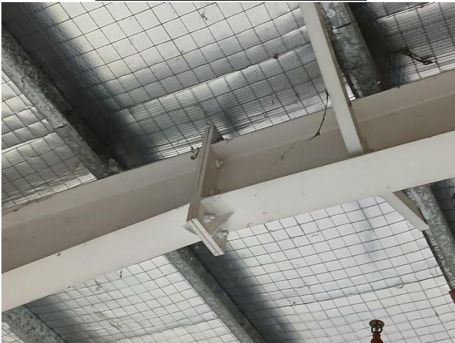
Typical rafter framing System
