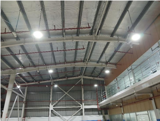
Typical rafter framing System
