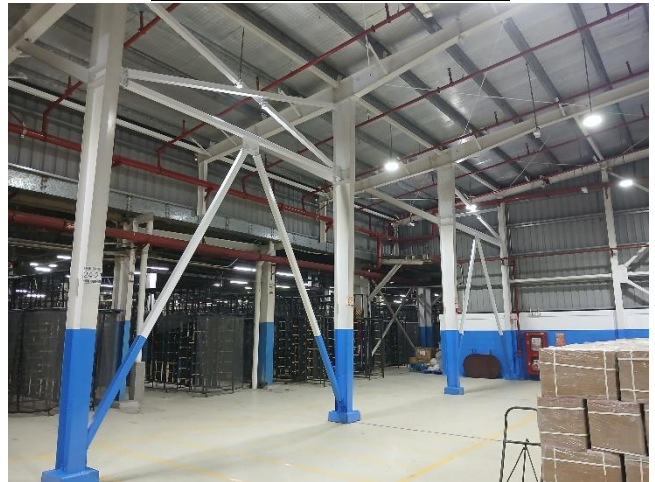
Steel beam column framing
