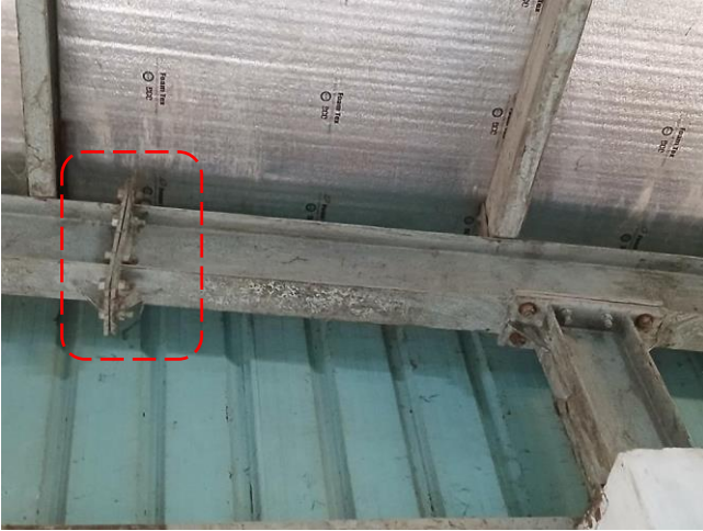
Improper connection and connection gap
