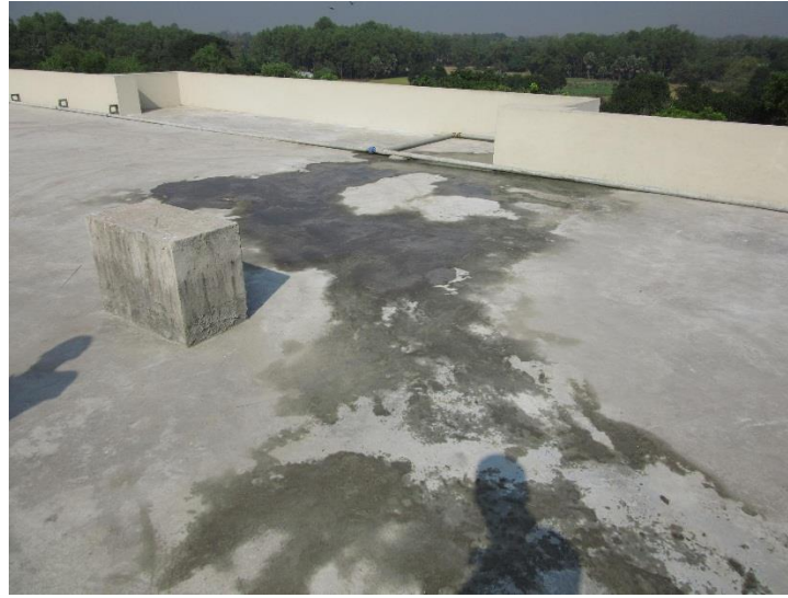
Water accumulation on roof slab
