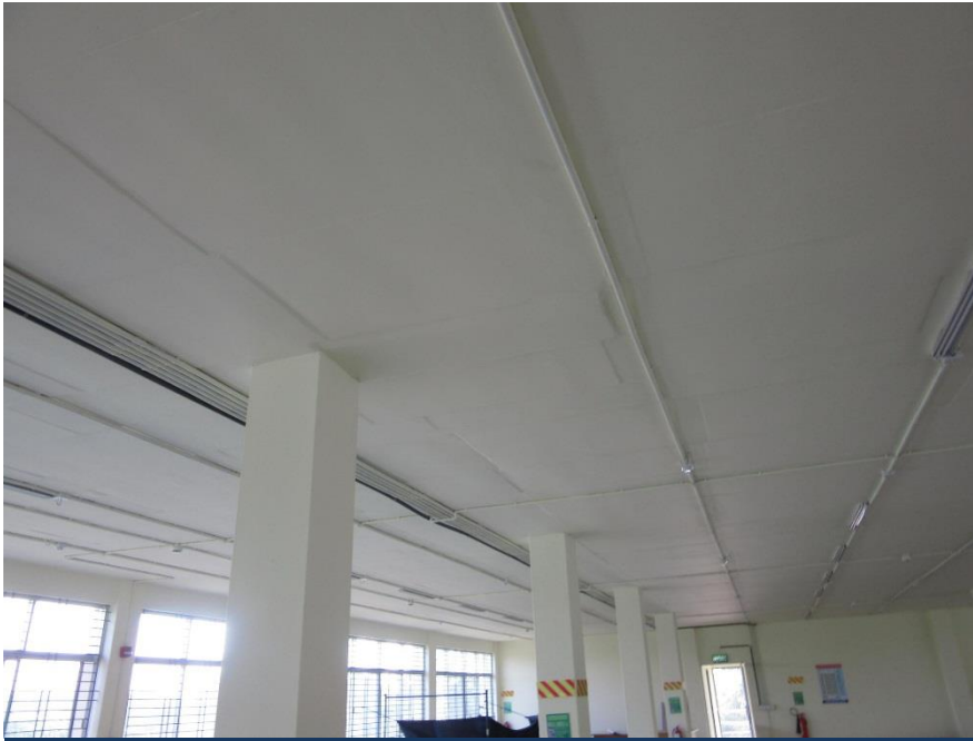
Flat slab without drop panels
