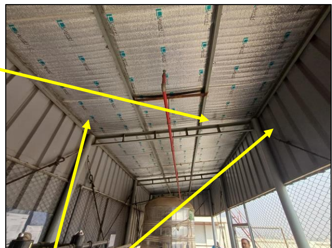
Roof bracing layout (RO plant)
