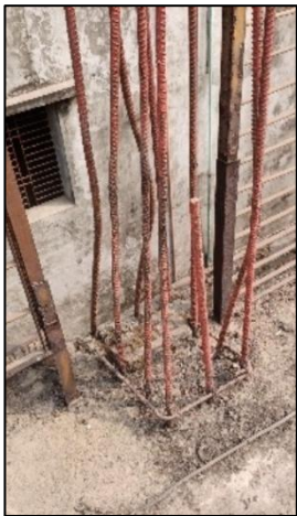
Column C1 (grid H-5) 10Ø16 re-bar found instead of 4Ø16+6Ø20
