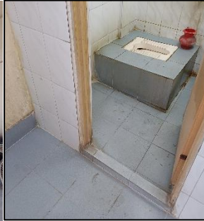
Floor and toilet built-ups were not mentioned in the drawing
