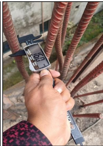
Column C1 (grid H-5) 10Ø16 re-bar found instead of 4Ø16+6Ø20
