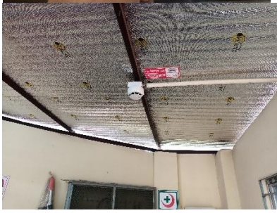
Member size and rafter layout not matched (Security Shed)
