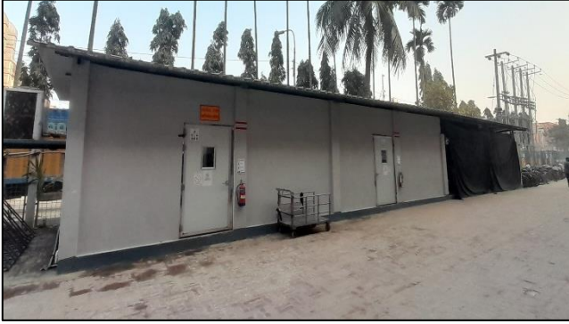
Chemical & Garbage Sorting Area
