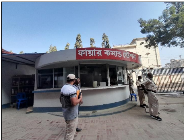
Security Post & Fire Command Station-2
