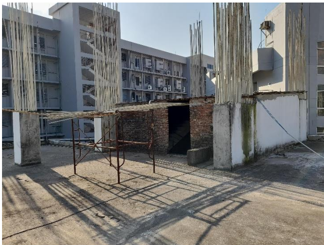
Steel truss roofing system
