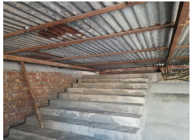
Truss angle rested on masonry wall
