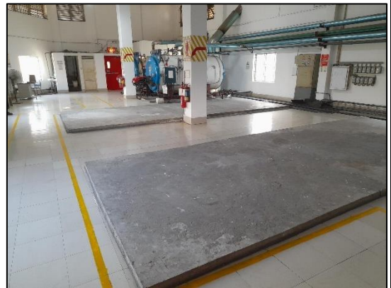
Existing buildup in ground floor
