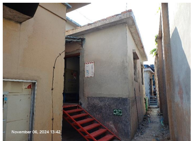
Stair of STP
