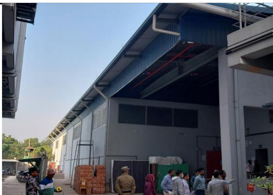
Building 6: Single Storied Fabric Store Shed (steel shed-9333sqfts)
