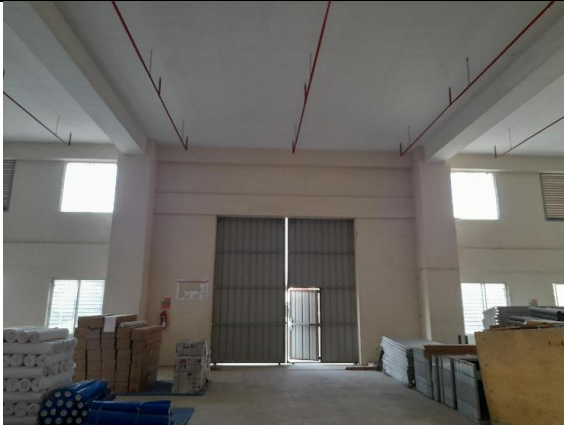
Tie beams with different levels
