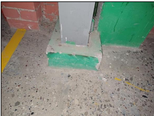
Columns are susceptible to trolley impact
