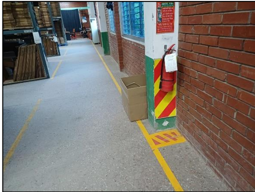
Columns are susceptible to trolley impact
