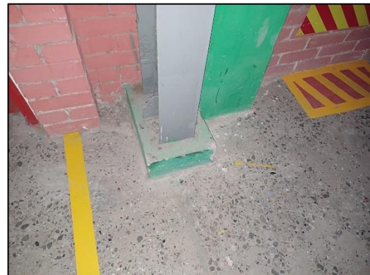
Columns are susceptible to trolley impact
