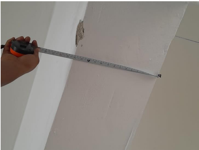
RB1 was measured as 350x475 mm which was shown as 300x475 mm in the drawing
