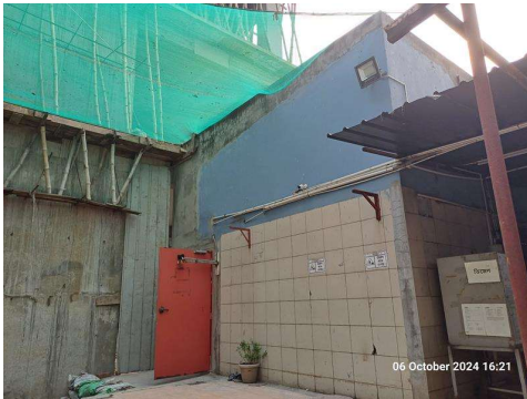
Building# 5- Boiler Room
