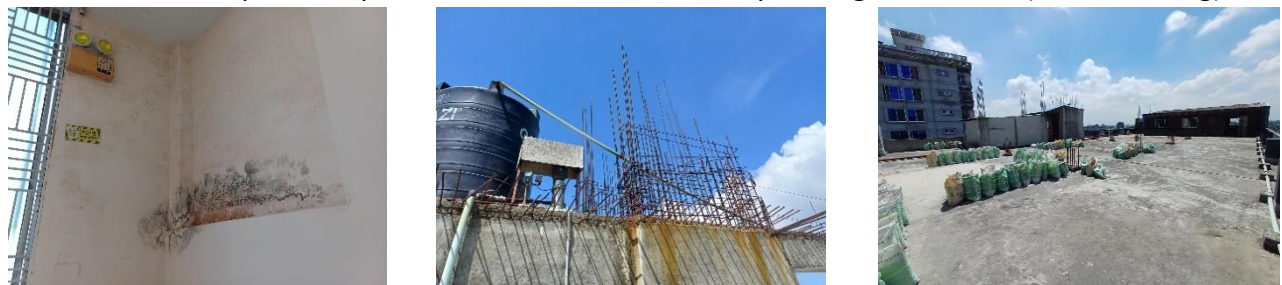
No waterproofing layer on the roof (MCAC on Roof)
