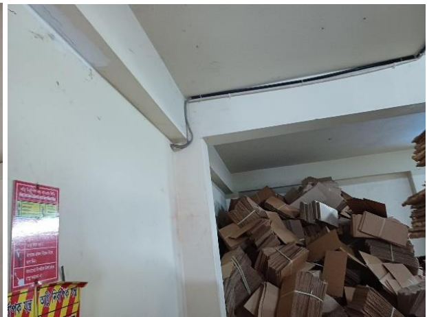
RC Beam-Column framing
