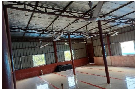
Steel Roof Shed (G+2 RC including steel roof shed)
