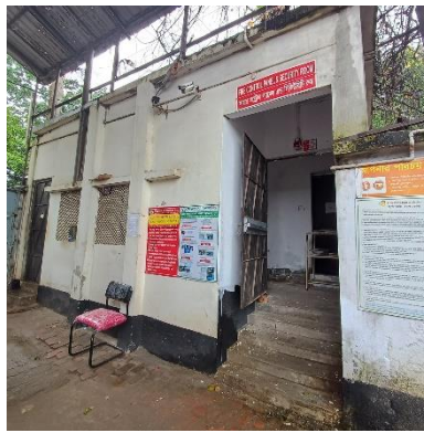
Fire Control Room
