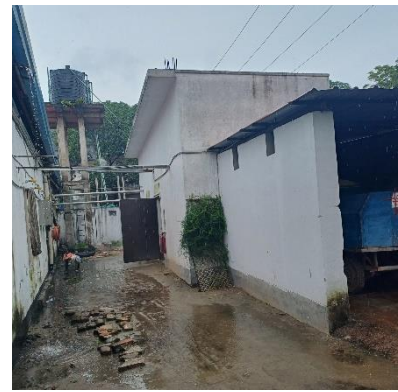
Boiler & Compressor Building
