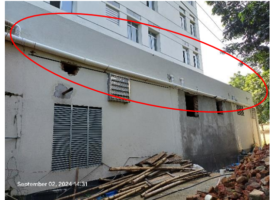
Utility portion columns only ground level
