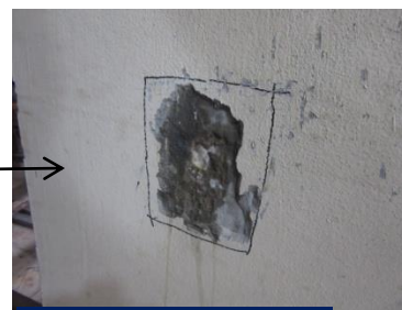
Internal Column (Stone)
