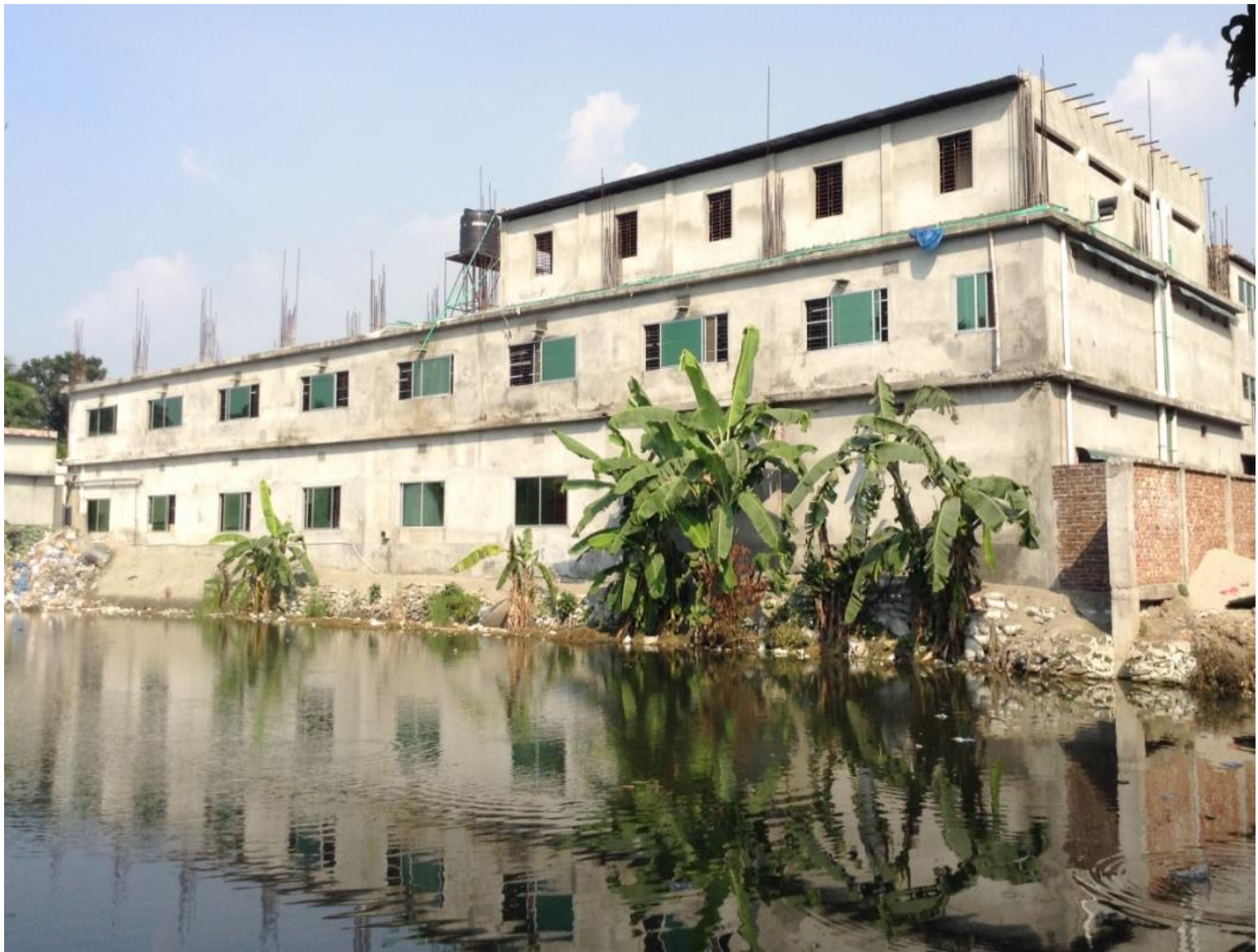
Water pond adjacent to the building.
