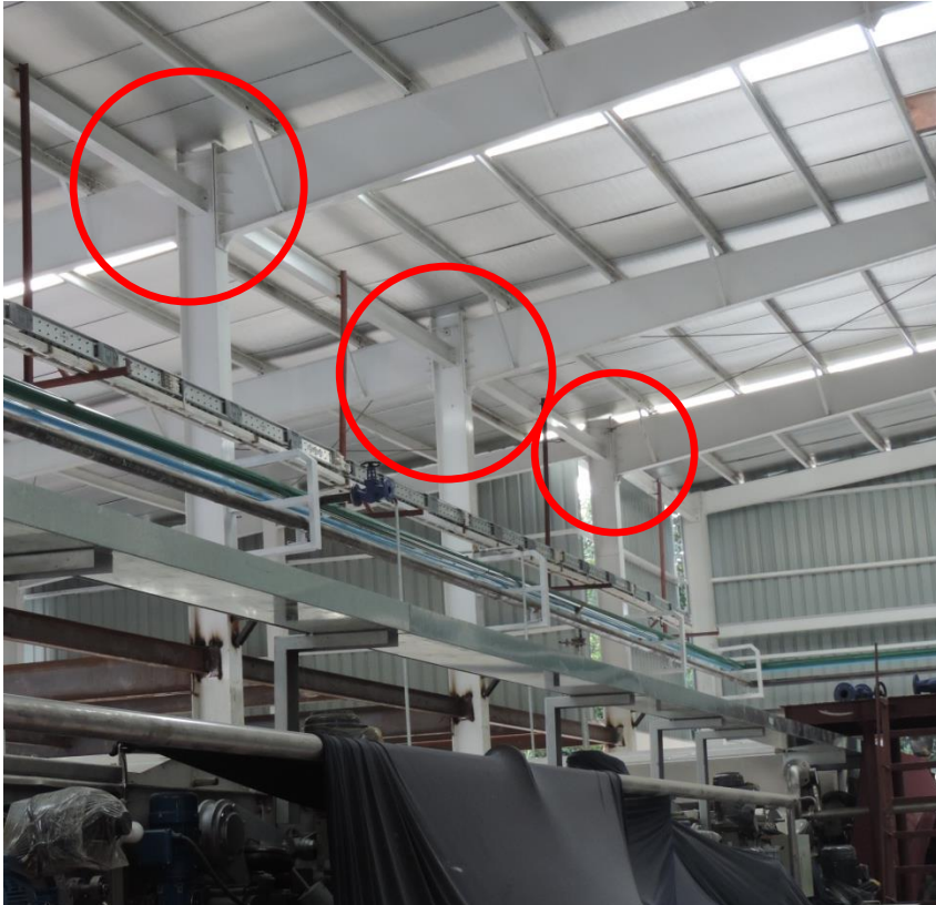
Portal 2 to 5 have no moment connection with column. (ability to act as a portal)
