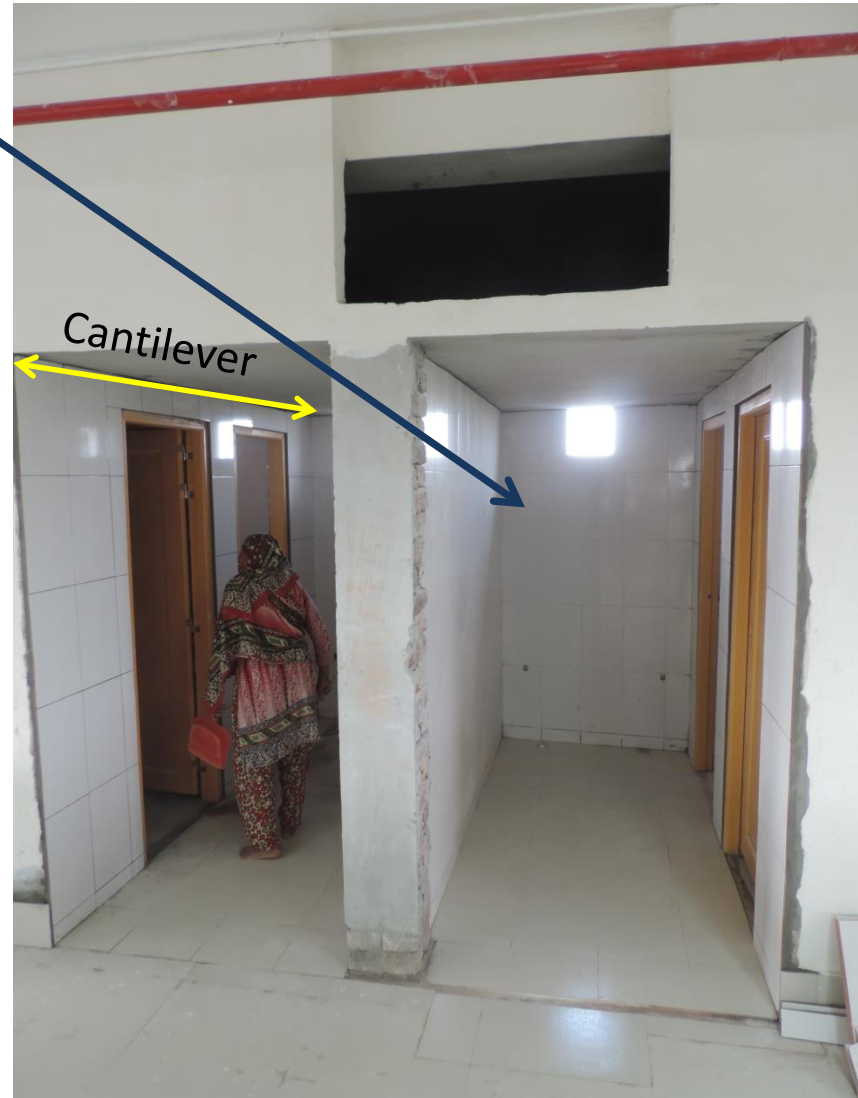
Toilets are on cantilever
