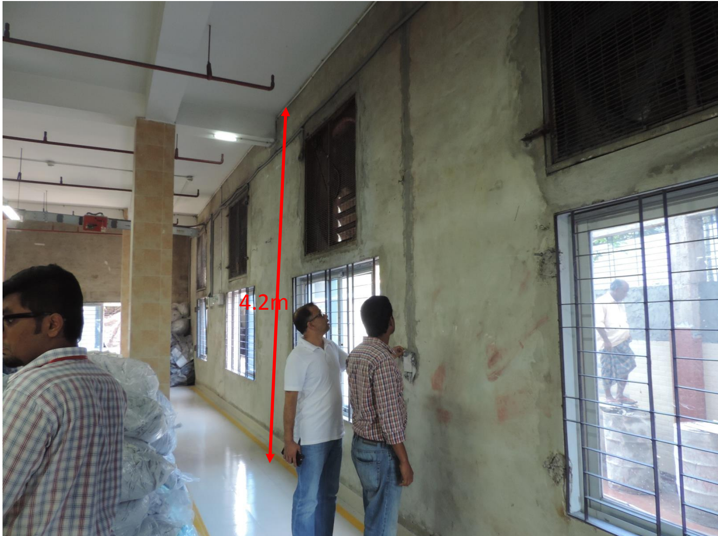
Ground floor large wall panels appear to be slender
