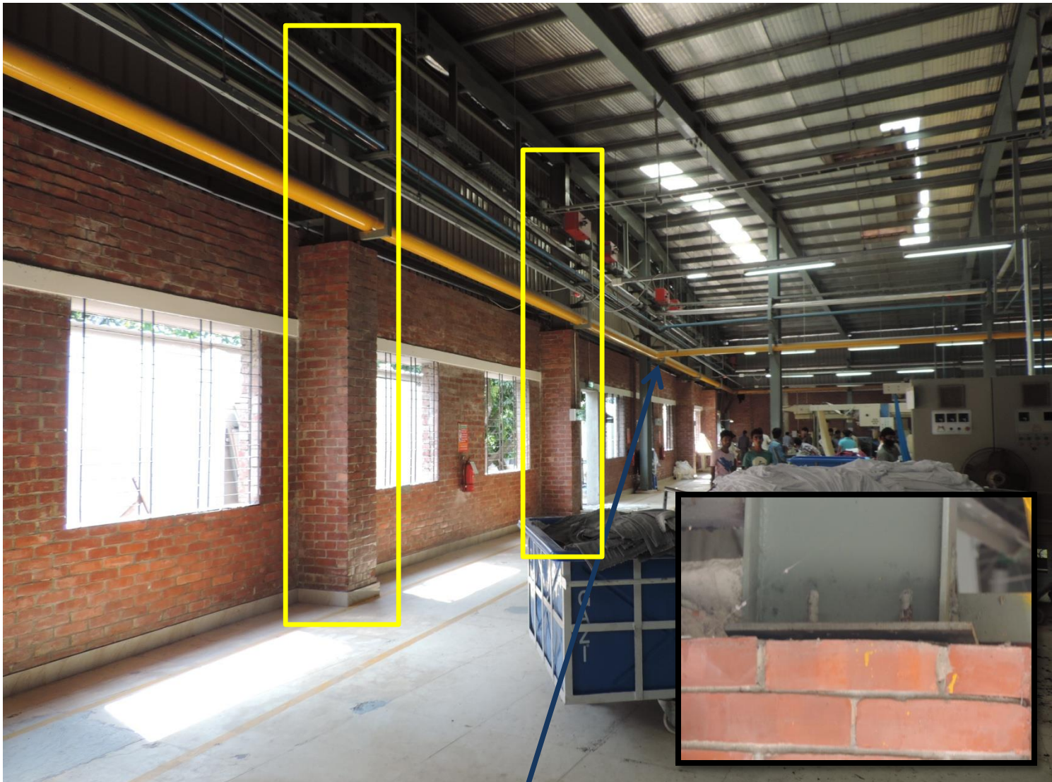
Gable columns constructed half height in concrete
