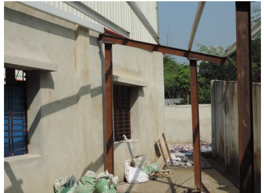
Non Engineered lean-too structure under construction as add-on to main shed
