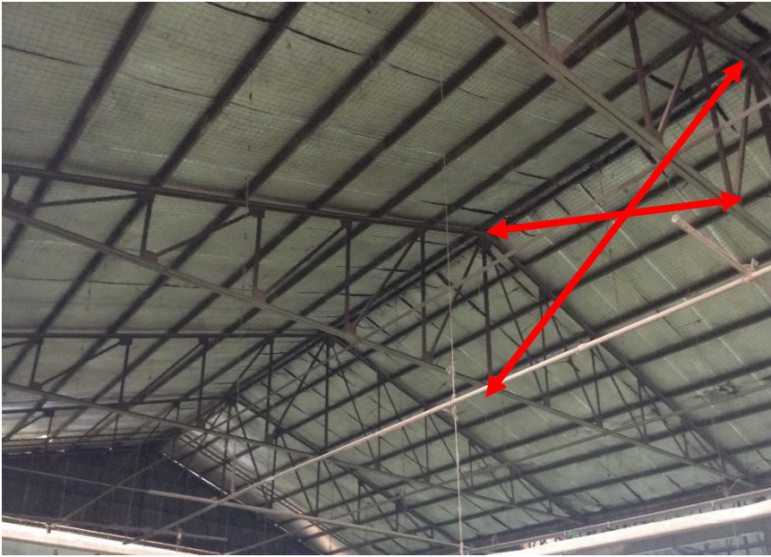
Lack of Vertical and Horizontal Bracing on Main Production Shed
