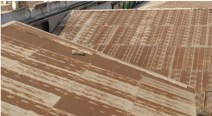
Poor Roof Insulation and Corrosion on Roof
