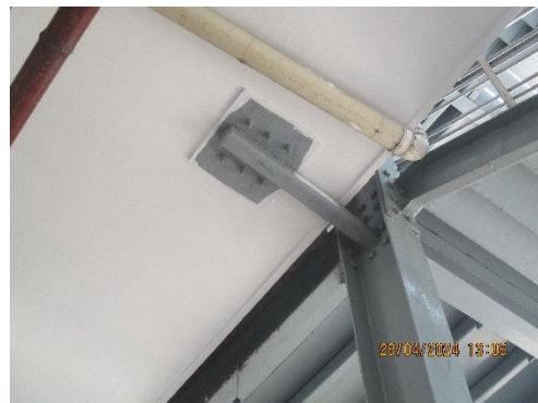
Connection with the main building
