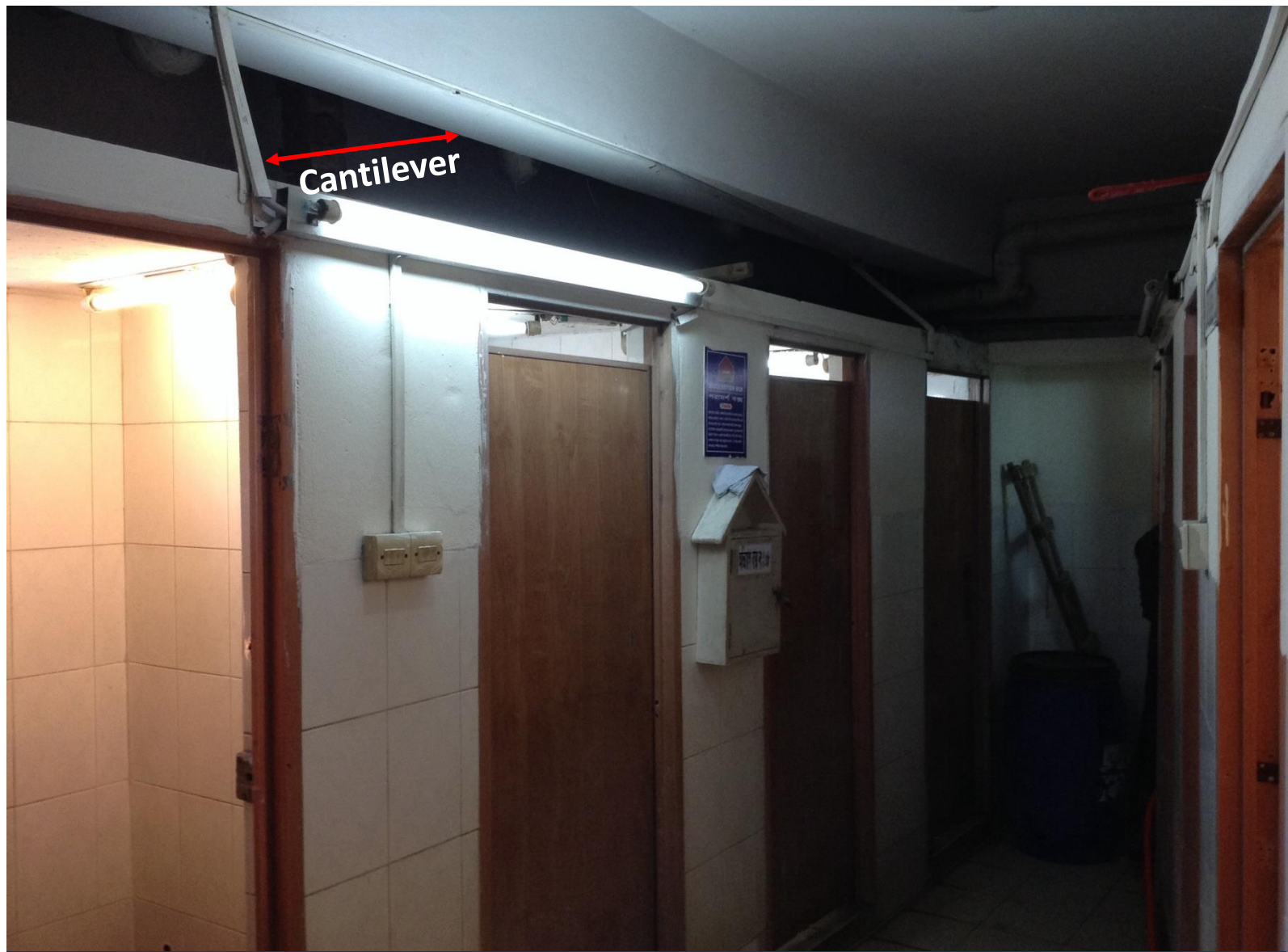
Toilets are on cantilever slab
